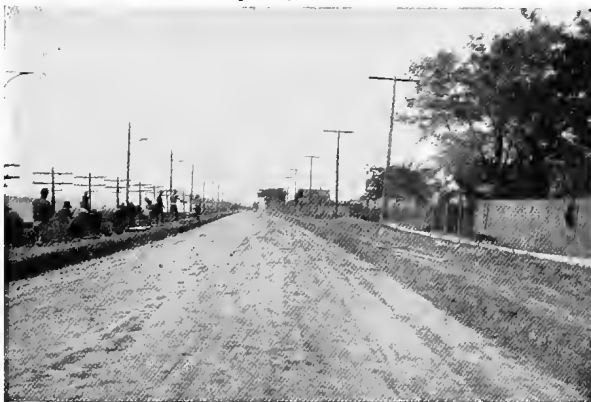
Finishing subgrade.
